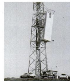
Big-scale demonstration of wireless power transmission by microwaves, scheduled for July and August 1975 by NASA's Jet Propulsion Laboratory and Raytheon, is readied at Goldstone, Calif. Dish antenna 85 feet in diameter (left foreground in photo above) will radiate 300 to 400 kilowatts toward a 12-by-14-foot receiver ("rectenna") a mile away on a hilltop tower, seen in right background of large photo and in close-up view at near right. It will recover sizable portion, expected to reach tens of kilowatts, of the beam. Pairs of high-intensity indicator lamps (far right) arranged in same pattern as rectenna's 17 elements, show which are energized as powerful beam sweeps across its target.
